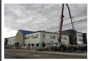
We're looking forward to moving families into The Meadowlark this spring! This month there's been a lot of progress on the outside of the building and the construction site. Siding is now mostly complete; all that remains is the orange painting on the front of the building. Solar panels will soon be installed. And the parking lot is being paved.
