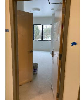
have doors up (pictured here). Lights inside of the rooms have been installed, and the private bathrooms are being tiled and finished up.
